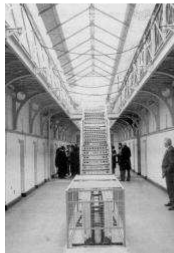
Military Detention Barracks
